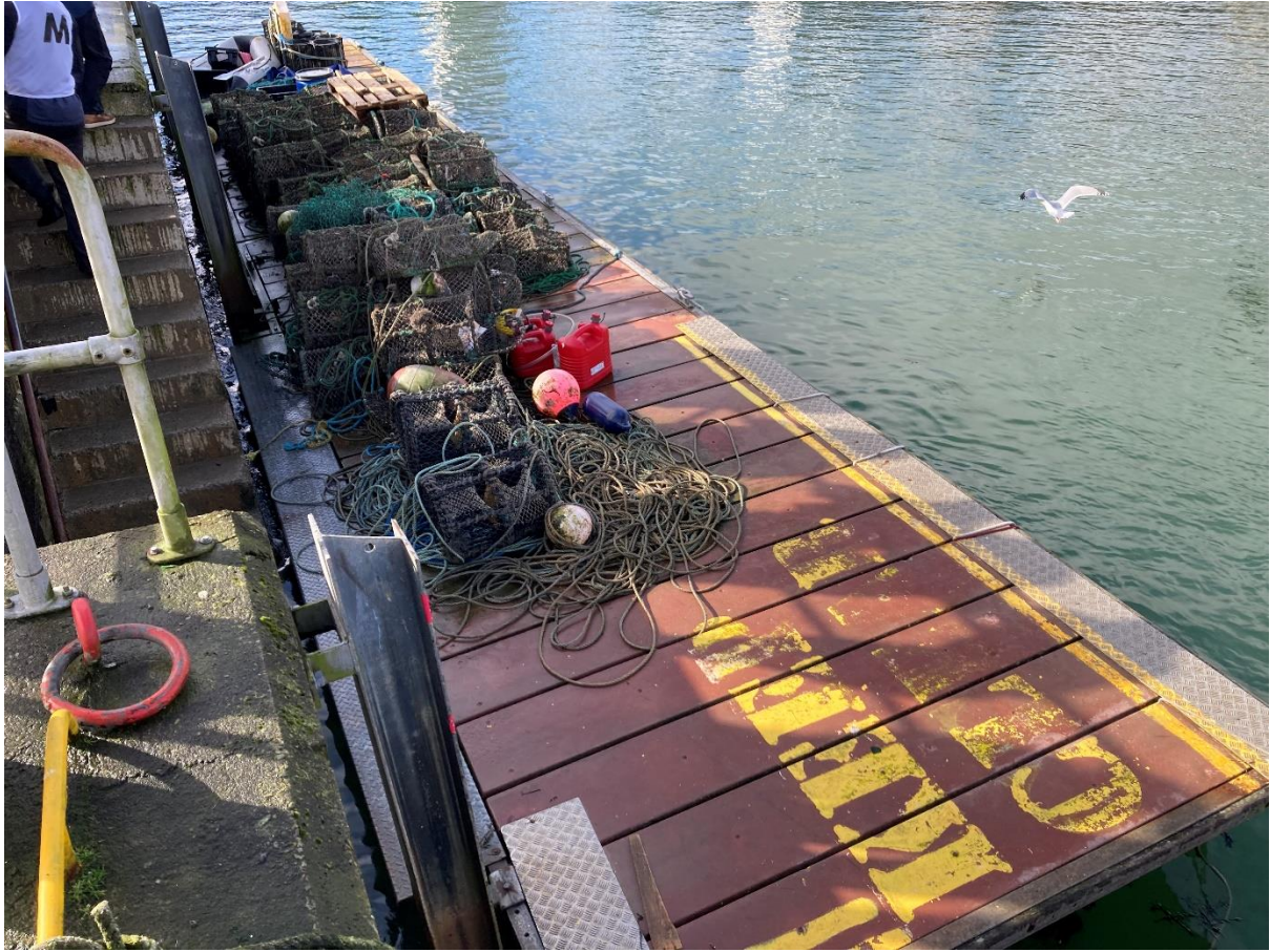
Figure 2. Photograph showing the pontoon in Schull Harbour.
